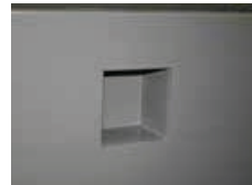
Cast-in Accessory Pocket. Insert light housing. Finished product.
