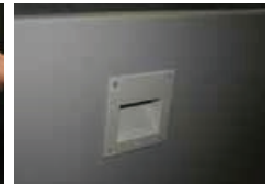
Cast-in Accessory Pocket. Insert light housing. Finished product.
